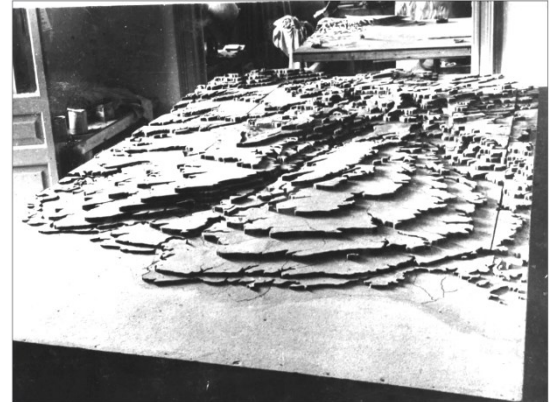
Figure 1. Hardboard contours nailed together and mounted in position at MEIU, Cairo. [Reproduced with kind permission of the Public Record Office.]
